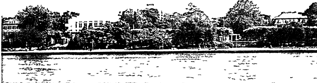
1. The new Museum für Kunsthandwerk, Frankfurt-am-Main seen across the River Main with the Schaumainkai beneath the trees. The old Villa Metzler on the left and the Museum für Volkerkunde on the right established the axis on which Richard Meier's new building is established
